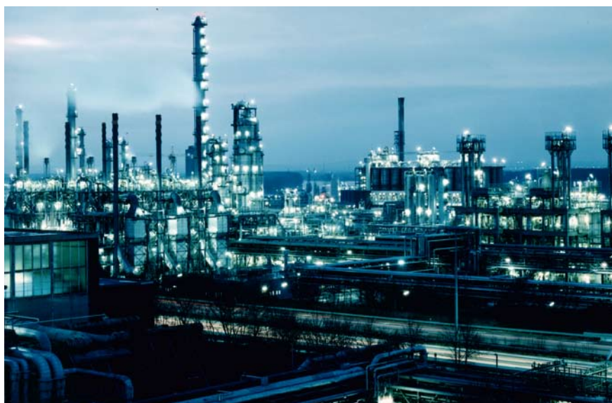
The Wesseling, Germany, complex is LyondellBasell's largest manufacturing facility in Europe
