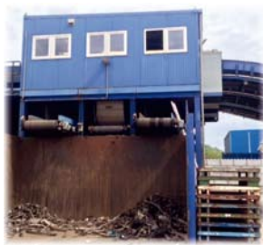
Ventilation & Venting for Sorting Cabins
