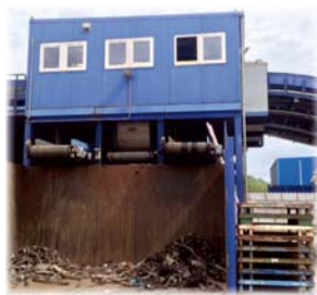
Ventilation & Venting for Sorting Cabins
