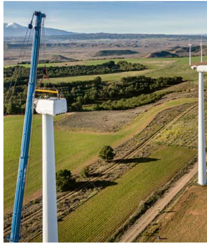
Old turbines being dismantled in the Montes de Cierzo wind farm
