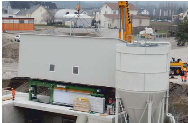
Strabag, Bürglen, Switzerland – Details of filter-press installation and housing
