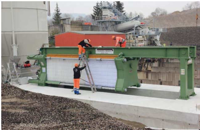
Strabag, Bürglen, Switzerland – Details of filter-press installation and housing
