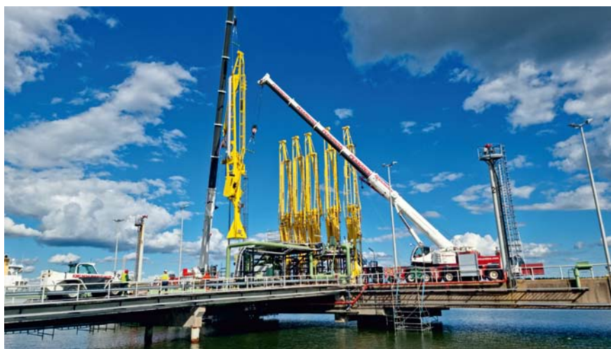
Installation of new unloading arm for liquefied recycled raw materials at Neste Porvoo refinery harbor, Finland
