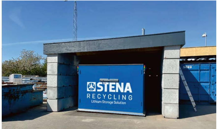
Stena Recycling Battery Center in Farum Denmark
